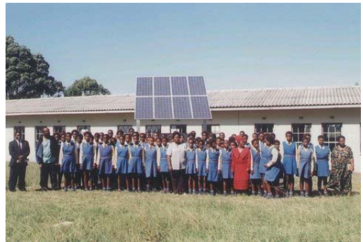
Example of solar electrification of schools (photo with courtesy of EPIA )
